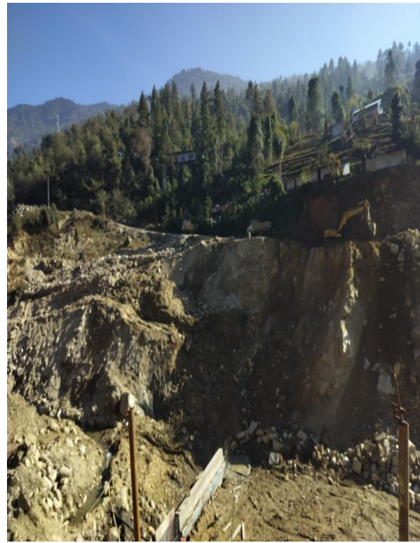
Left Bank Cracks at Headworks
