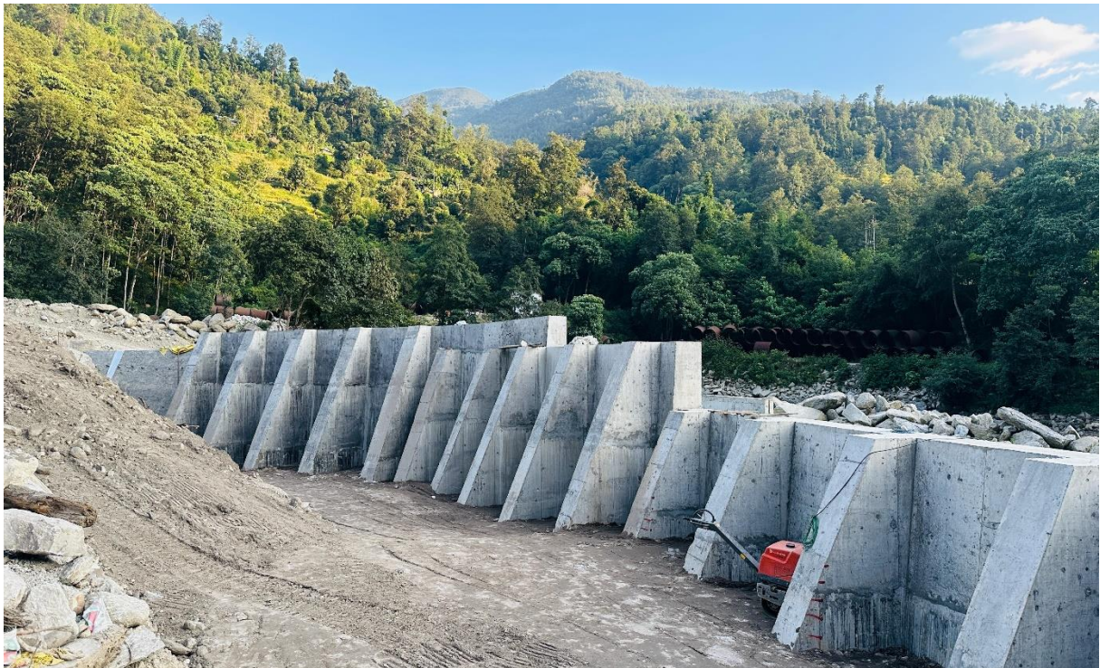
Switchyard Retaining Wall
