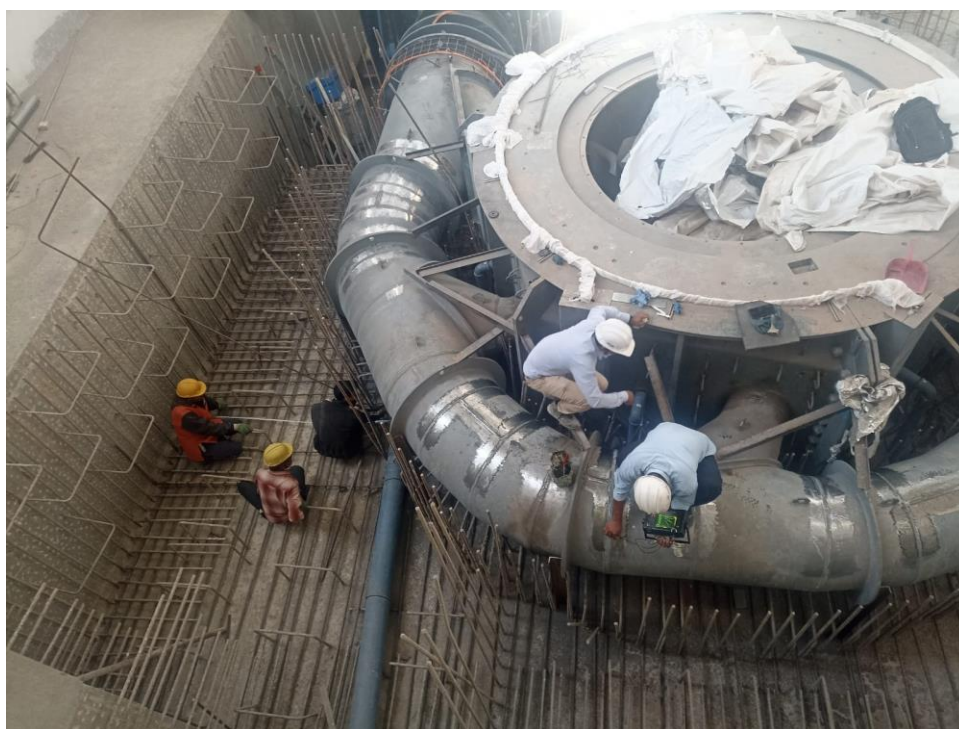
UT test of distributary pipe Unit 3
