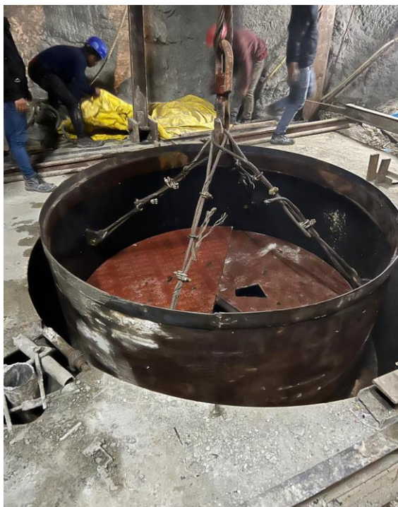
Penstock Pipe Lowering at VS-1
