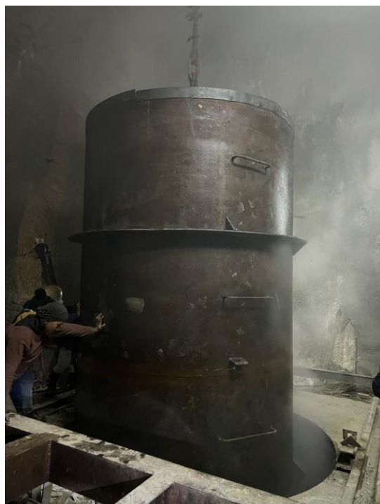
Penstock Pipe Lowering at VS-1
