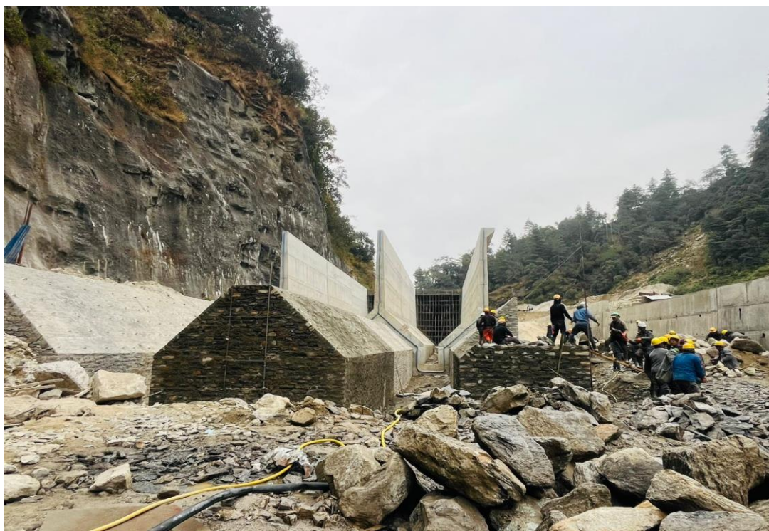
Settling basin (masonry wall)
