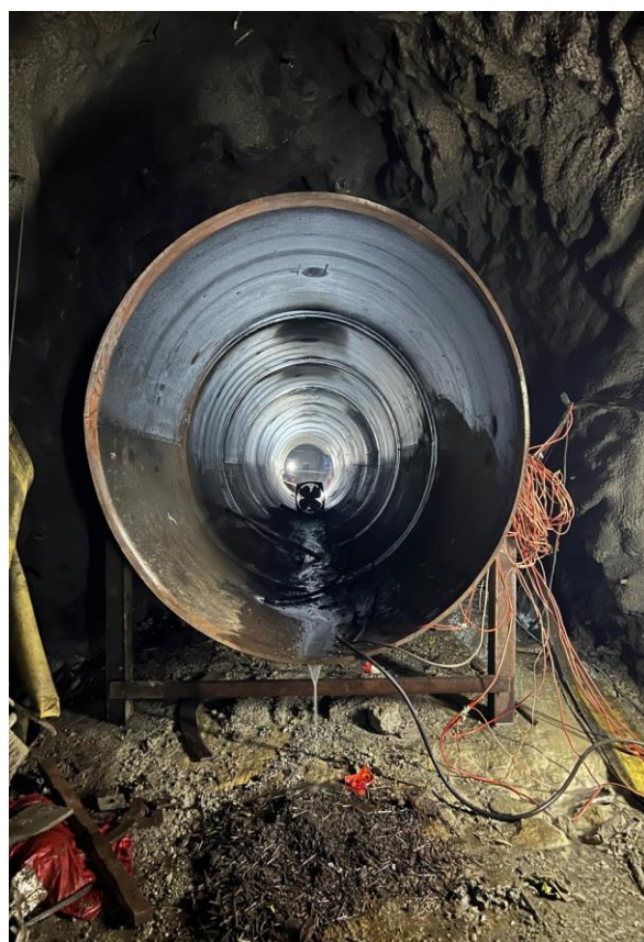
UPT Pipe Erection
