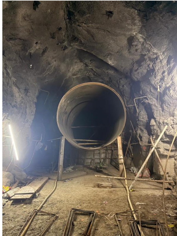
Pipe Erection at Surge
