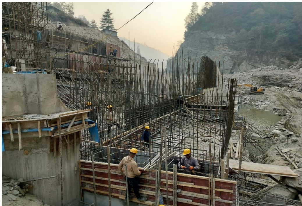
Ogee weir rebar and formwork
