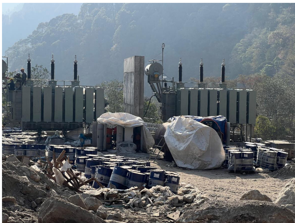
Installation of Power Transformers
