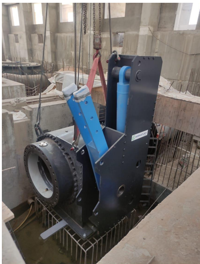
Installation of Unit 3 MIV
