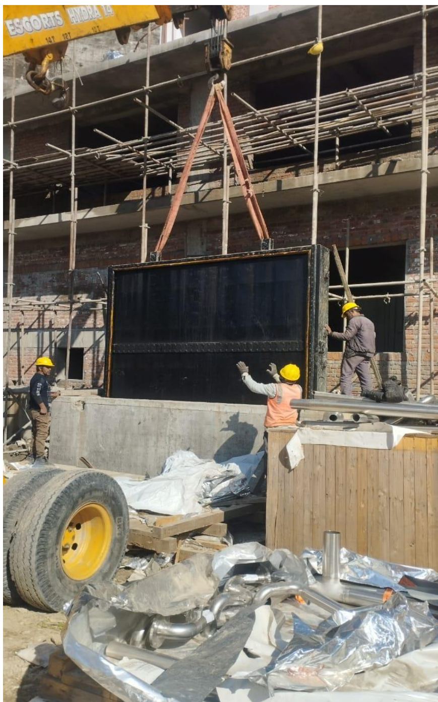
Dry Testing of Turbine Outlet Gate
