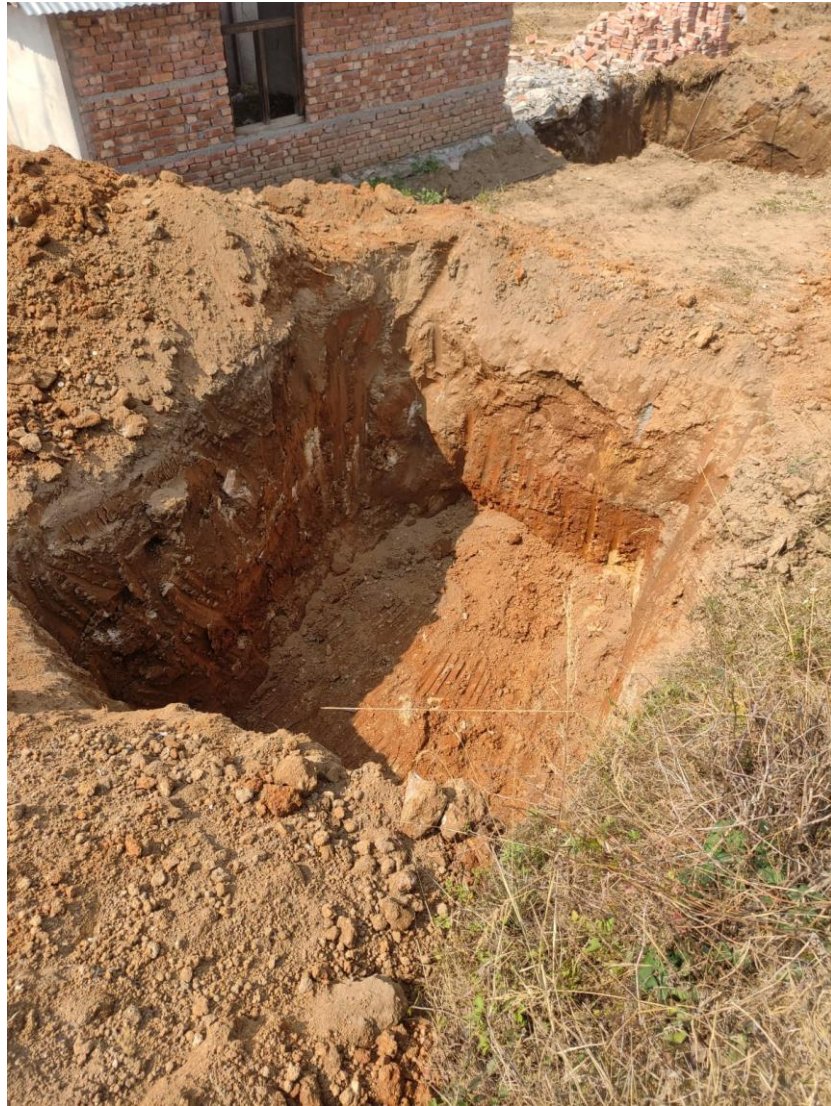
AP 6 foundation excavation works
