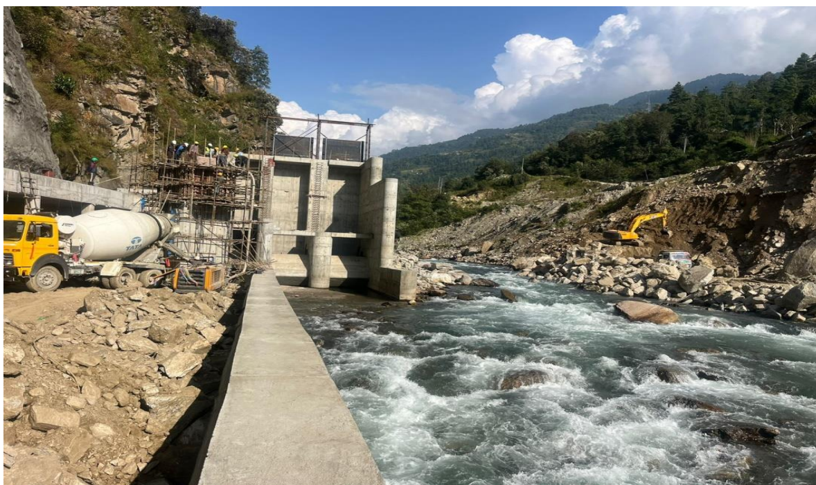
Headworks Undersluice
