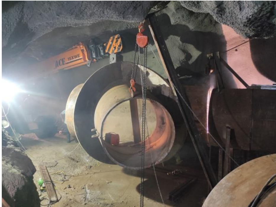
Bifurcation-I Erection Works
