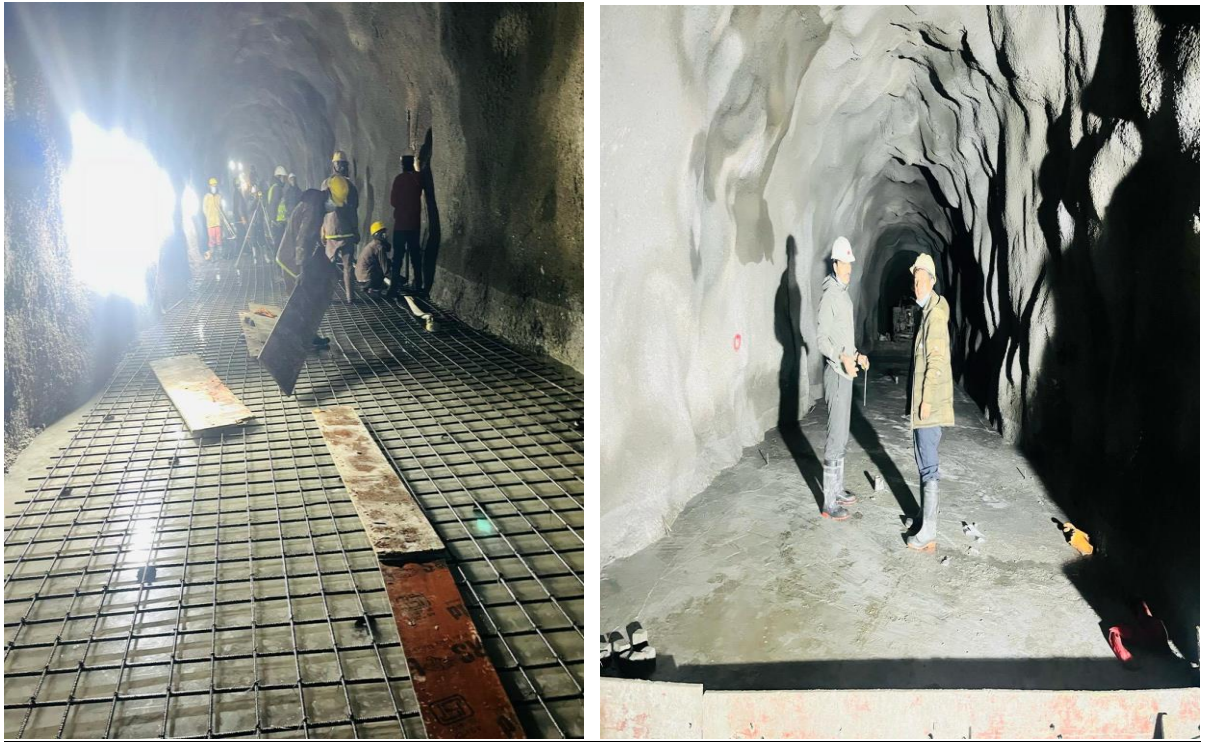
Inlet Lining works
